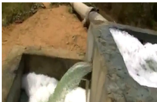
Figure 1(b). Pumping of sewage water from nearby drainage channel.
